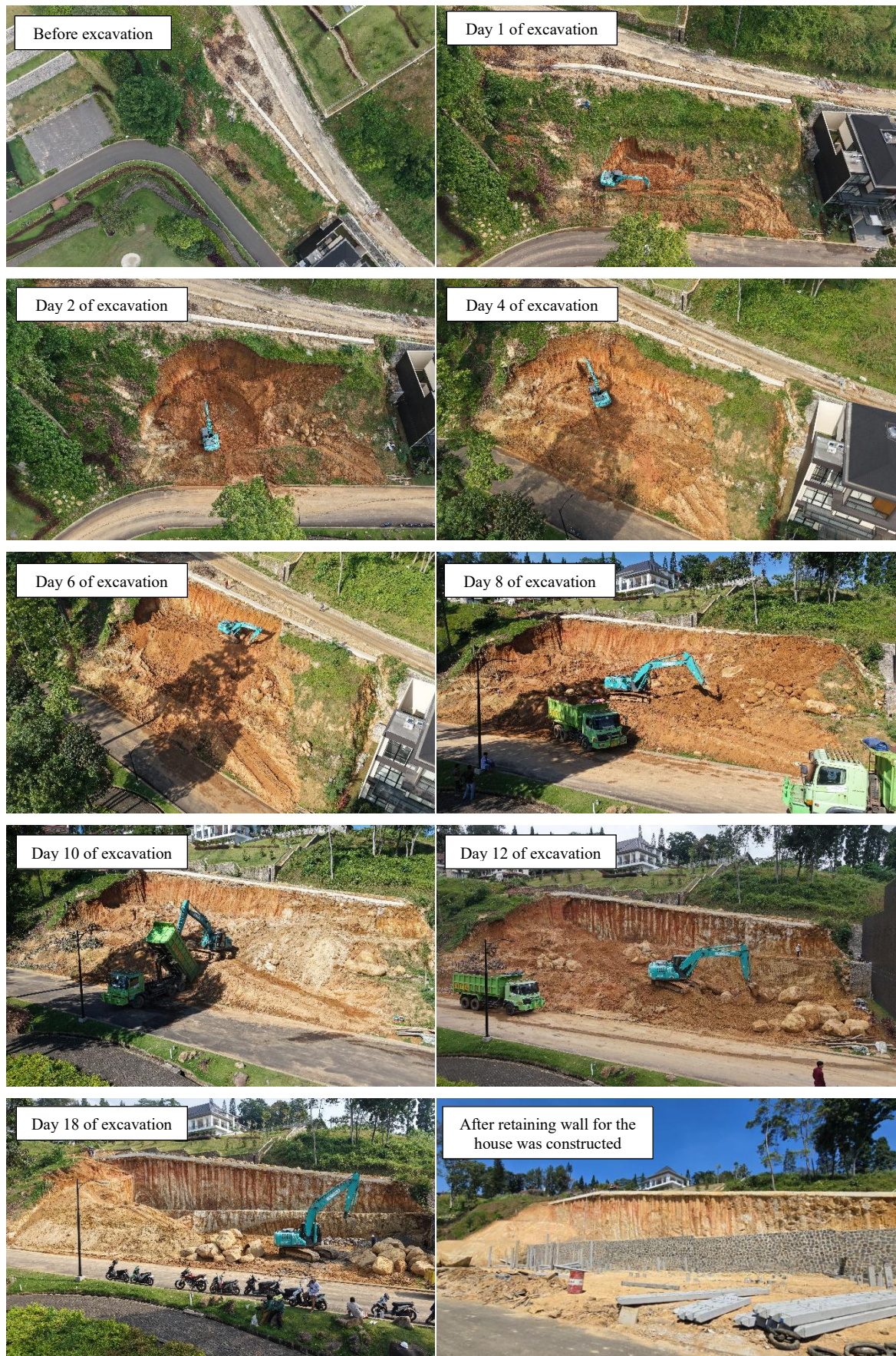
Figure 6. Photographs of the excavation at different stages
