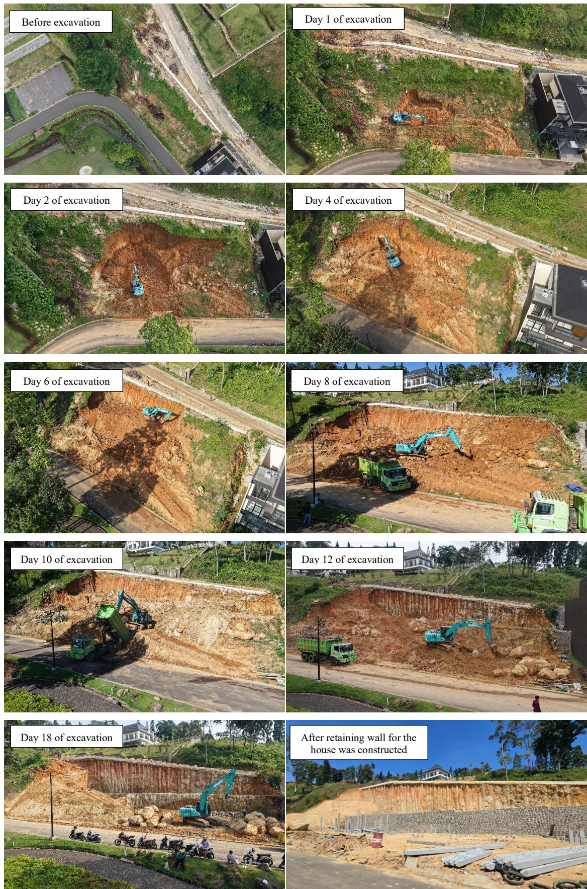
Figure 6. Photographs of the excavation at different stages
