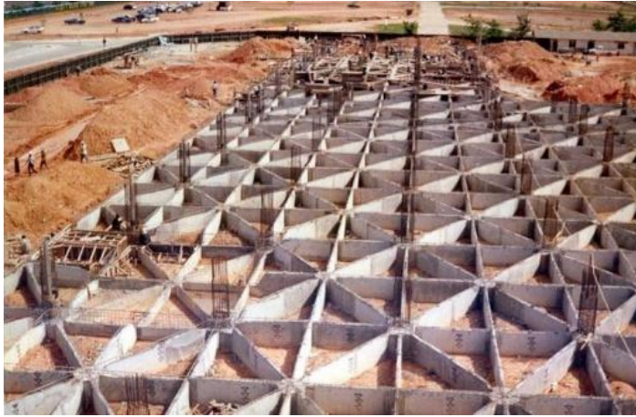
Figure 1. Illustration of KSSL / Spider Web Foundation (PT Katama Suryabumi, 2011)
