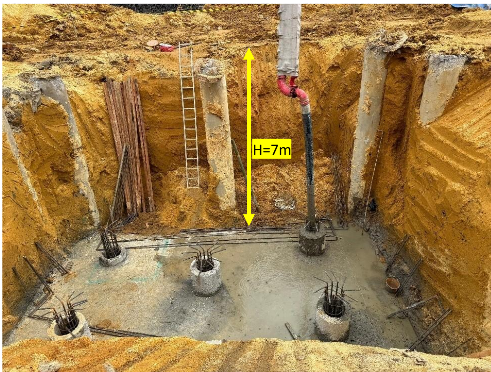
Figure 12. Example of deep excavation of residual soil
