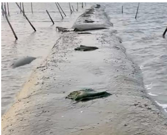
Figure 13. GI-Tube 2 years post-installation
