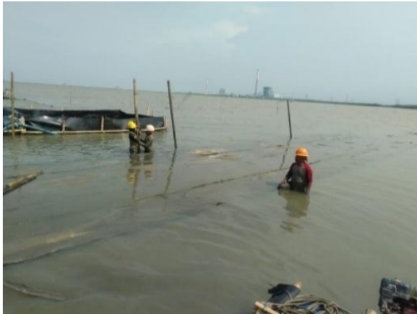
Figure 5. Bamboo piles installation
