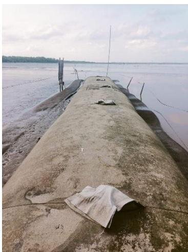
Figure 11. GI-Tube condition after 100 days
