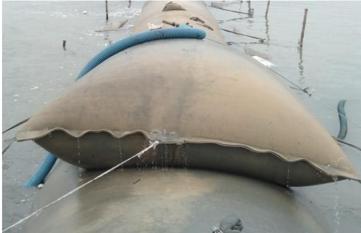
Figure 12. Clear water discharged from the GI-Tubes
