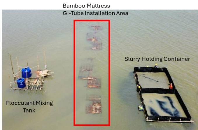
Figure 6. Layout of the construction area
