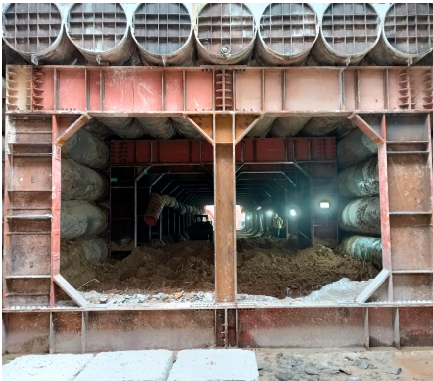
Figure 18. Photograph after the mining excavation work was completed.
