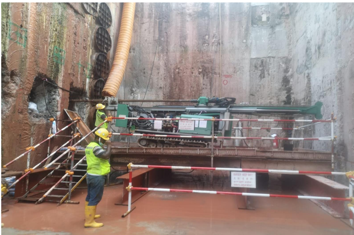
Figure 16. Photograph of horizontal grouting work.
