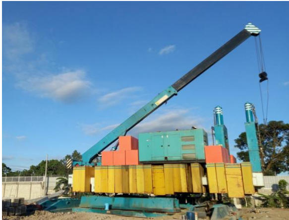
Figure 4. Hydraulic static pile driving rig in the Philippines (photo from author)
